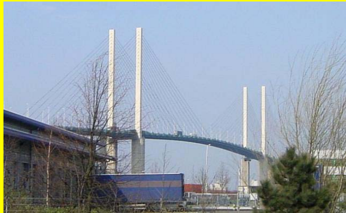
A photo of an Essex Landmark—The Dartford Crossing bridge—an example of the technical expertise that goes into designing and creating our built environment
